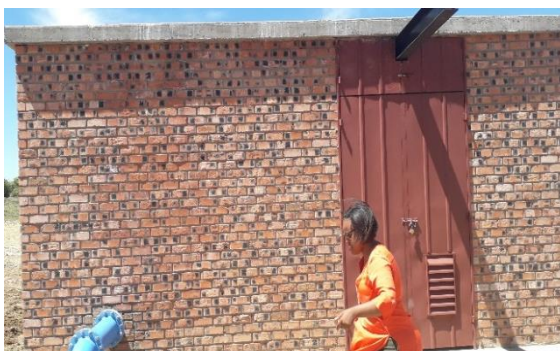
Figure 3: A photo showing the Sediba water pumping station
