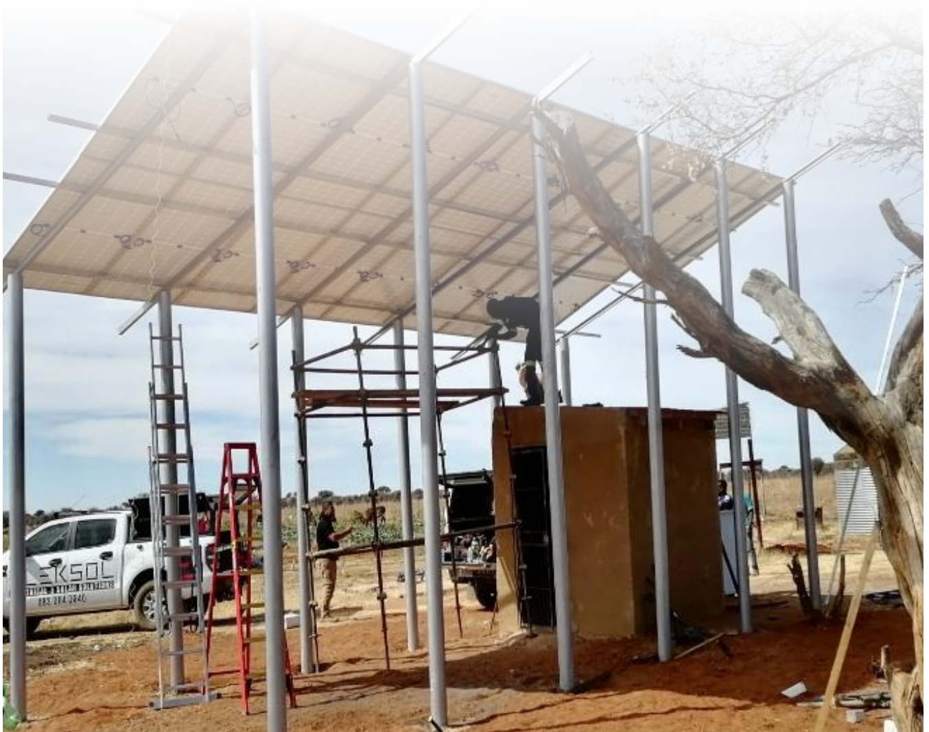
*A 10kW solar system that powers irrigation
